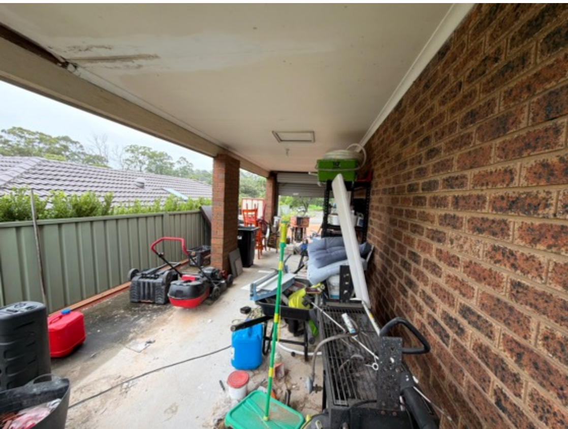
The garage area is in serviceable condition.
