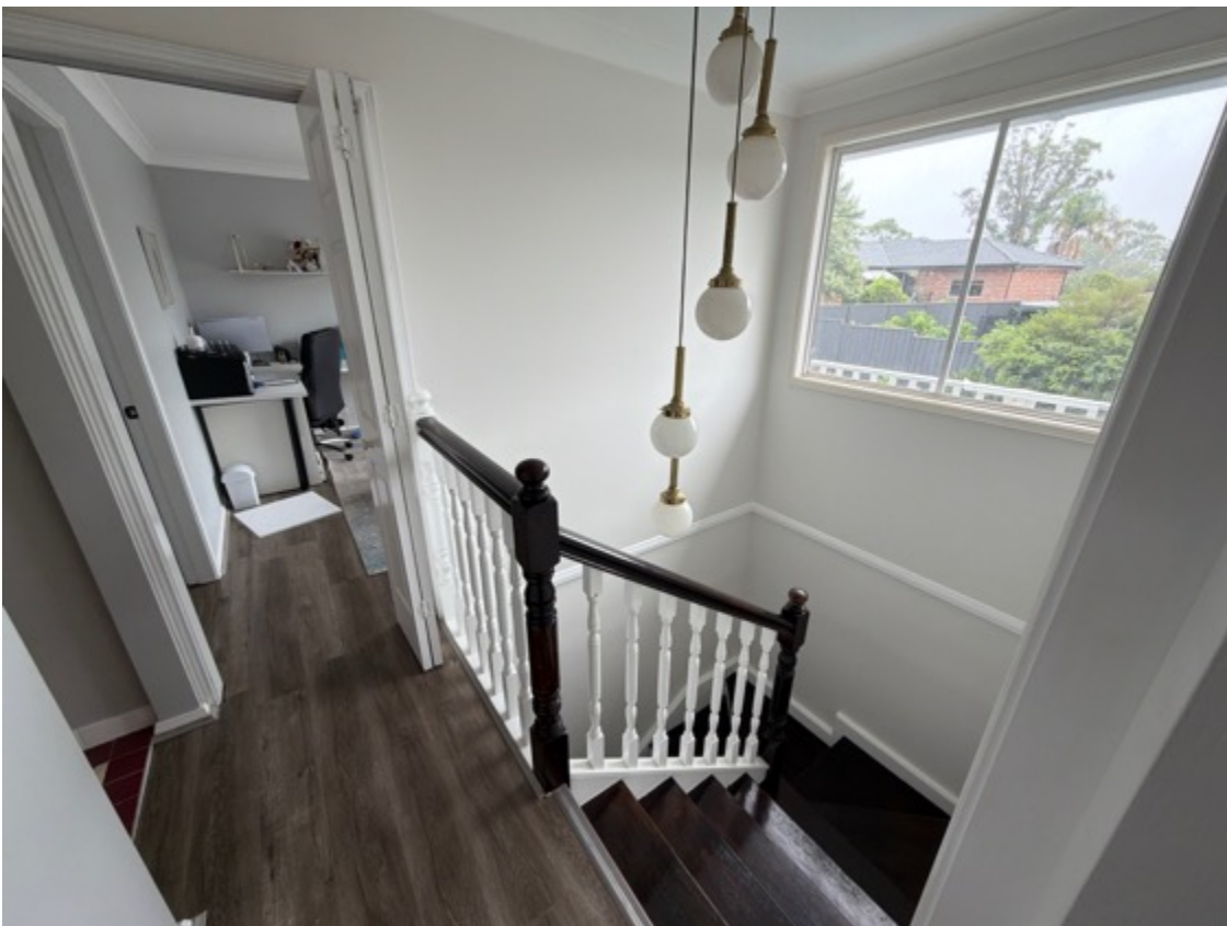
Interior railings checked are structurally sound.
