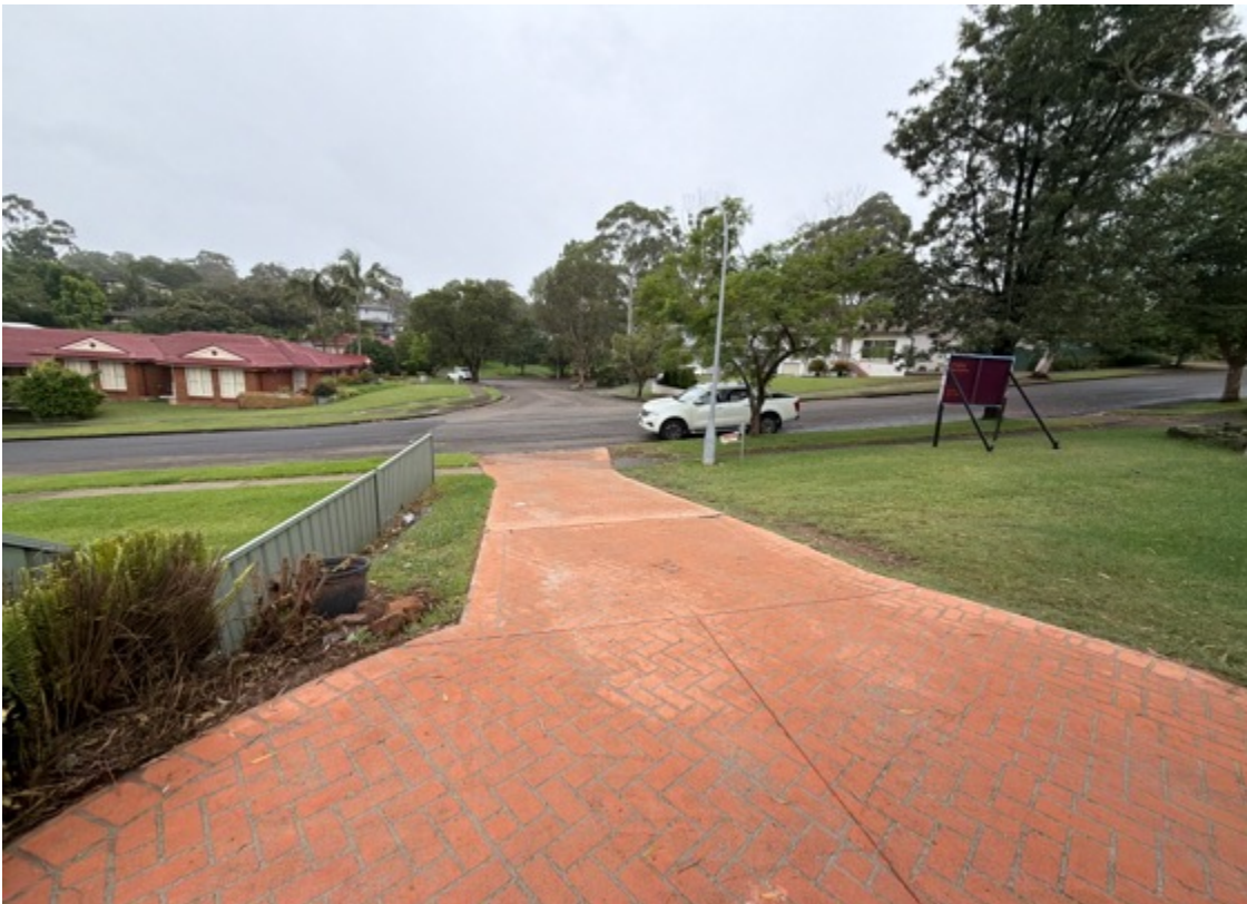
Isolated sections of exterior concrete displays typical shrinkage cracks and undulations - consistent with age.
