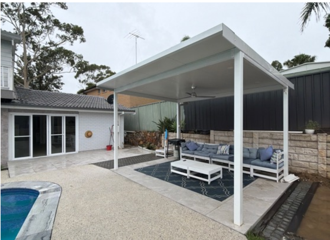
The rear pergola checked is structurally sound.
