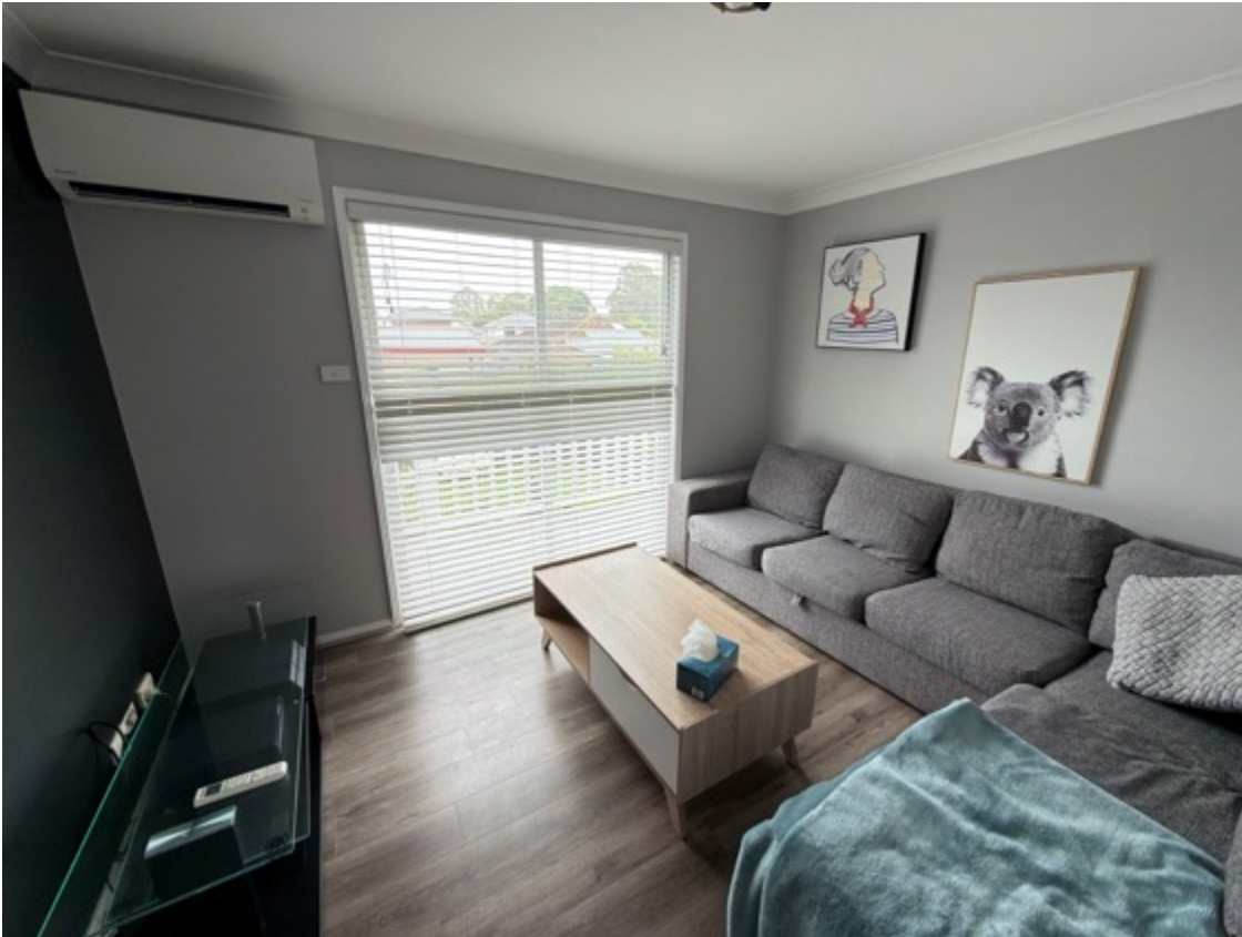
The wall mounted AC tested, functioned at the time of inspection.
