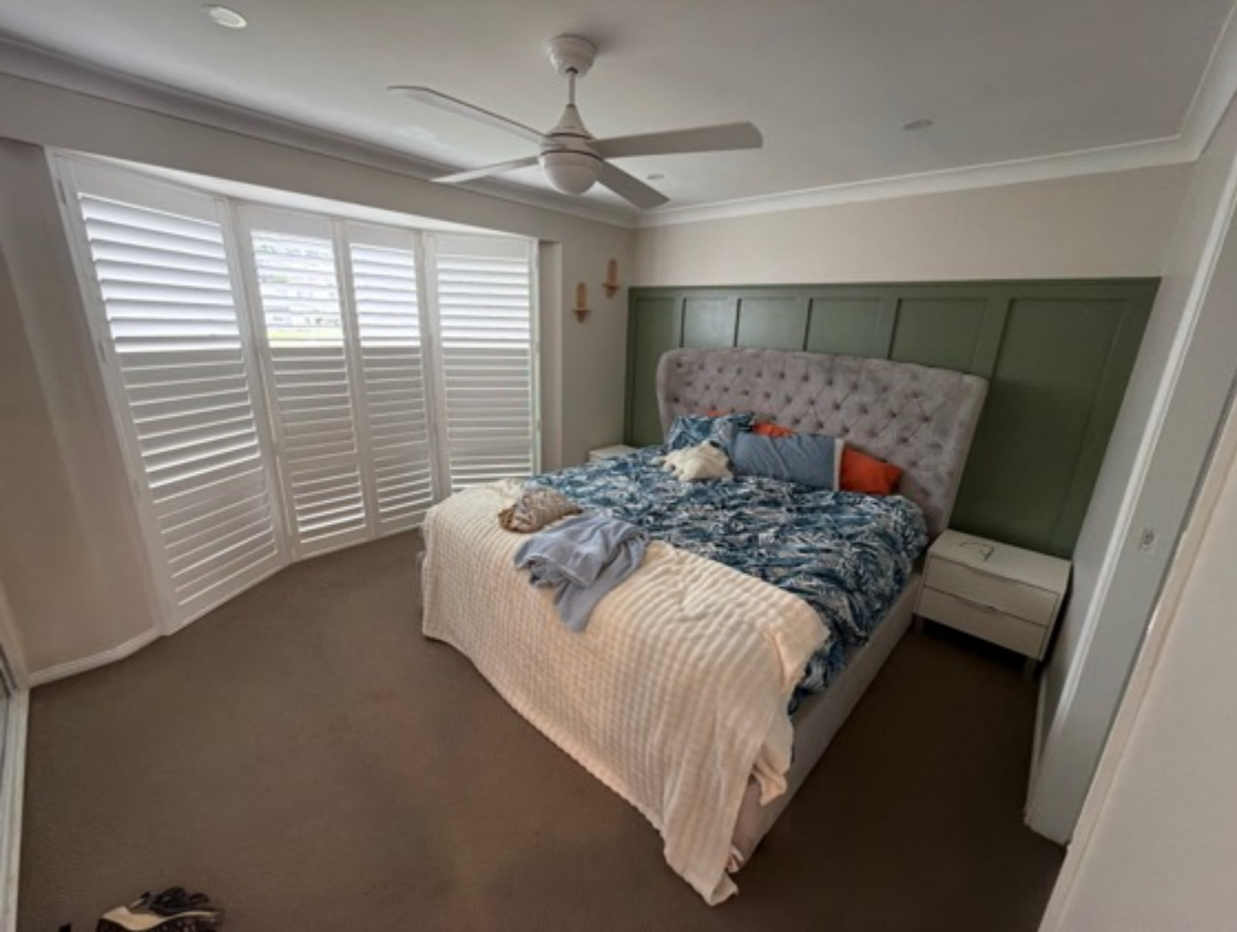
The main bedroom area presents in satisfactory condition for the age.
