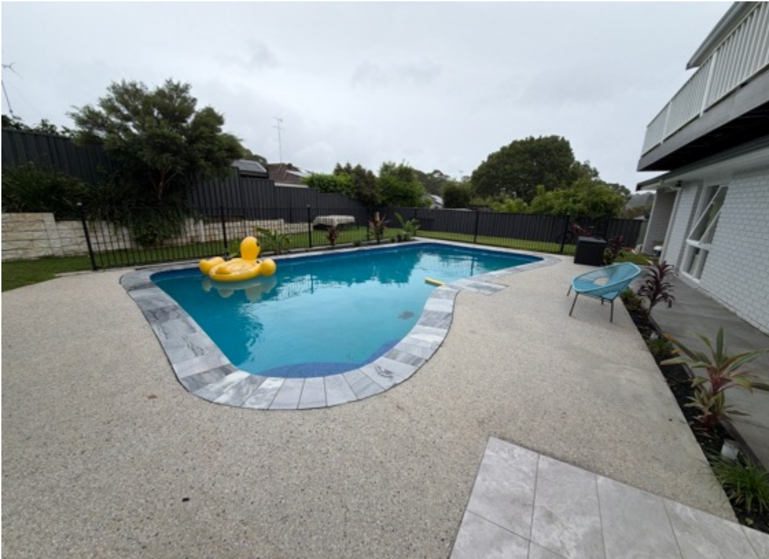
The pool area presents in satisfactory condition for the age.
