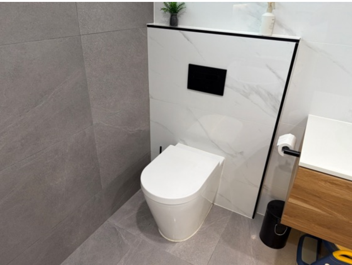
The toilet tested, functioned at the time of inspection.
